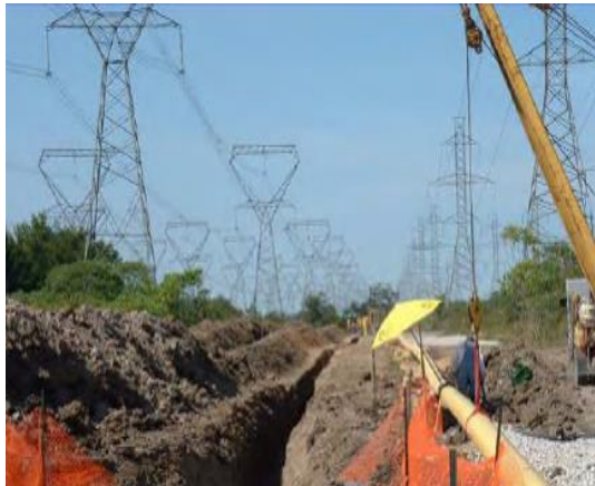
serious interference to the buried steel pipeline nearby
